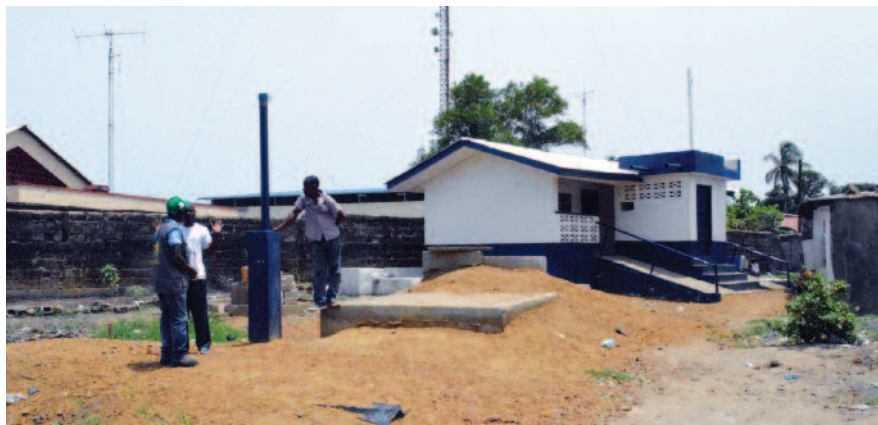
The photo shows the full site including latrine building, bio-digester and well, Zondo Town, Monrovia, Liberia. From left to right: William W. Slewro ,WASH Programme Manager, Concern, Dennis G. Letquiab, Chairman, Zondo Town Community, Albert Morris, CDO Construction, Concern. Photo by Sofie Johansen, 2015.
