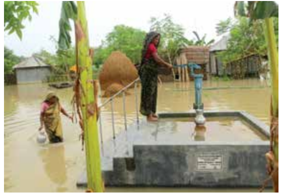
Shallow tube-wells with high platforms are installed to keep the water safe during floods. Photo: Concern Worldwide, Bangladesh
