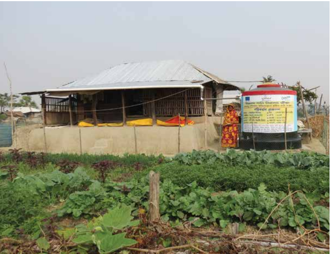
Participants are supported with rainwater harvesting systems and poly-bed vegetable gardens in their households so that they can produce enough vegetables to ensure their food and livelihood security. Photo: Concern Worldwide, Bangladesh
