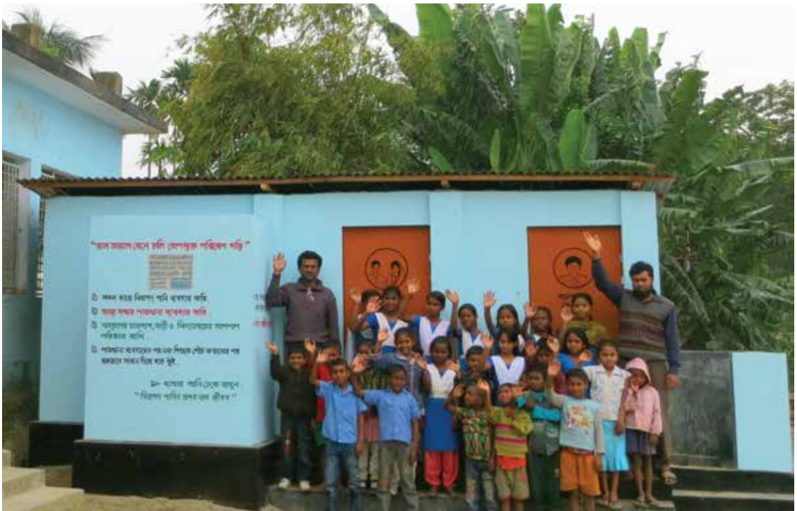
3-unit block latrines are constructed inside school compounds. Photo: Concern Worldwide, Bangladesh
